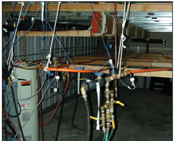
Figure 4. Test Rig for Uninsulated PEX-Al-PEX
